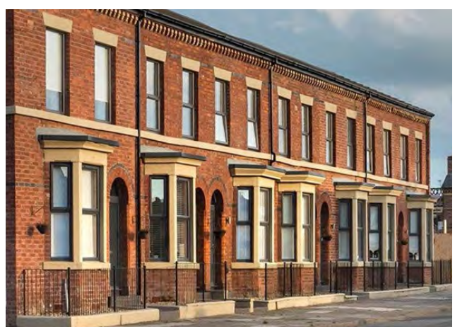
Figure 54 Refurbished Victorian terrace houses providing affordable family housing
