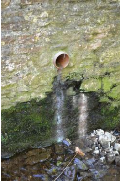
Figure 80: A 15cm diameter pipe located on the left bank wall of Keward Brook at survey point KB17. Note the prominent staining on the wall caused by the discharge of effluent from the pipe.
