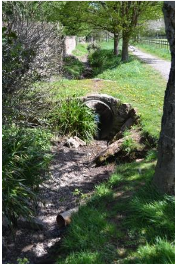
Figure 178: Upstream view of St. Thomas's Stream approximately 70m downstream of survey point ST8. A culvert and a 16cm diameter pipe (on the left bank) are visible.
