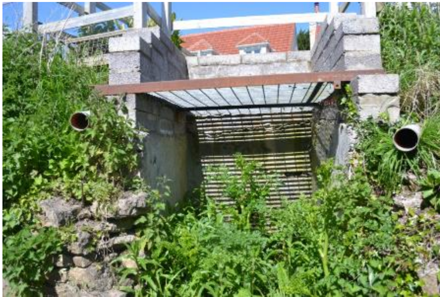
Figure 155: Two 10cm diameter discharge pipes and a single 20cm pipe (behind vegetation) on the left bank of St. Andrew's Stream approximately 65m downstream from survey point SA13. The purpose of the 10cm pipes in not known although a mild foul smelling dour was present.
