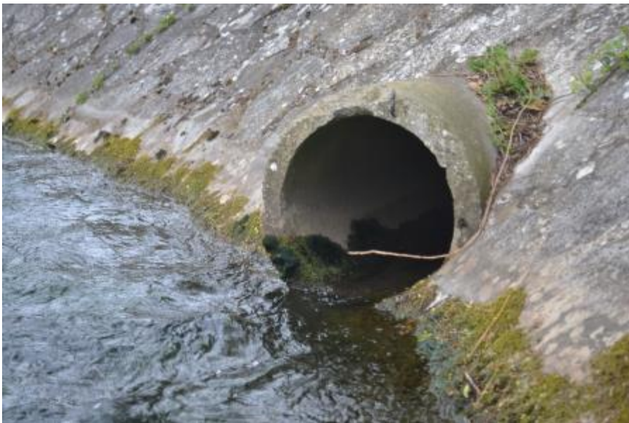
Figure 51: A 50cm diameter pipe, located on the left bank, discharging effluent into Keward Brook approximately 20m upstream of survey point KB11. The effluent was odourless and clear at the time this image was taken.
