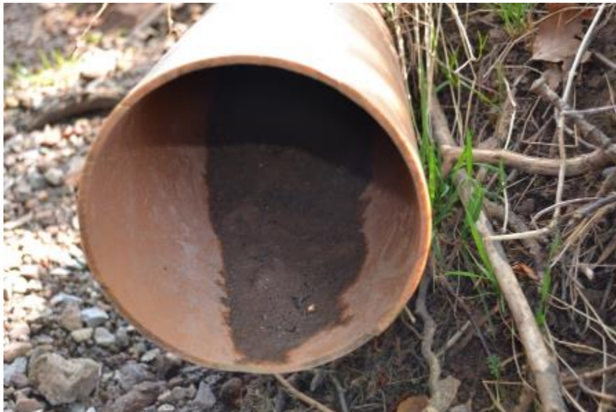
Figure 179: Close up image of sediment in a 16cm diameter pipe located approximately 70m downstream of survey point ST8. No effluent was being discharged and no odour was present
