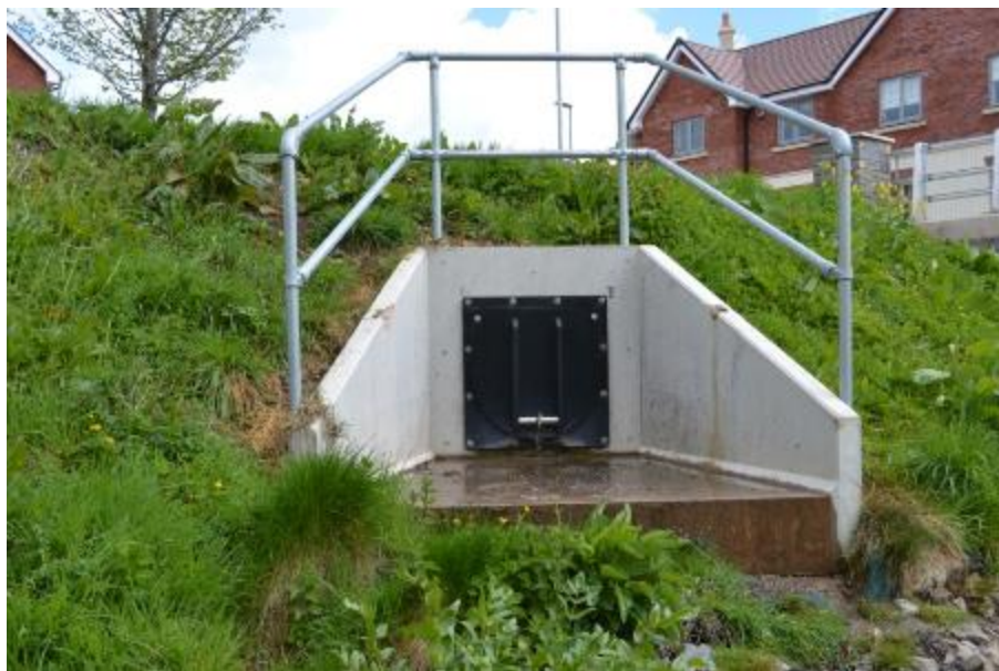
Figure 71: A 50cm diameter surface water drainage discharge pipe situated on the right bank of Keward Brook, approximately 80 m downstream of survey point KB15.
