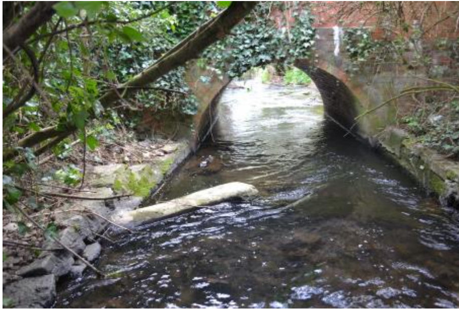
Figure 26: Downstream view of the third bridge located downstream of survey point KB5. Note the downstream facing concrete groyne on the left bank.
