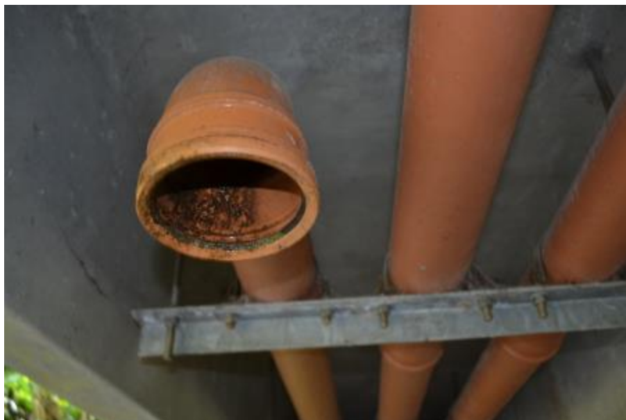
Figure 25: Pipe under the first bridge located downstream of survey point KB5. The 15cm diameter pipe runs from the left bank and dispenses directly into Keward Brook. No odour was present, although brown residue can be clearly visible close to the exit.
