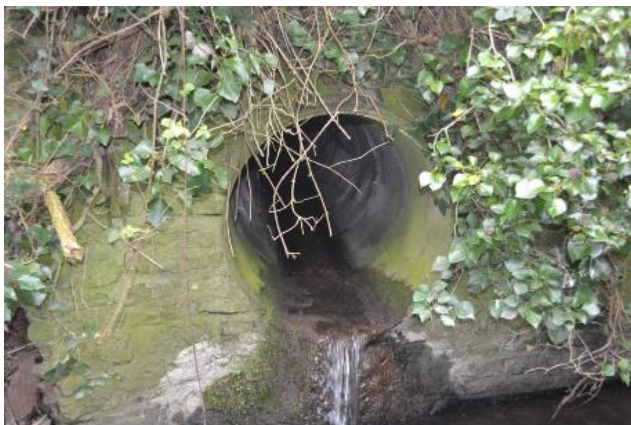
Figure 56: A 90cm diameter pipe, located on the left bank, discharging effluent into Keward Brook approximately 75m downstream of survey point KB11. The effluent was odourless and clear at the time this image was taken.
