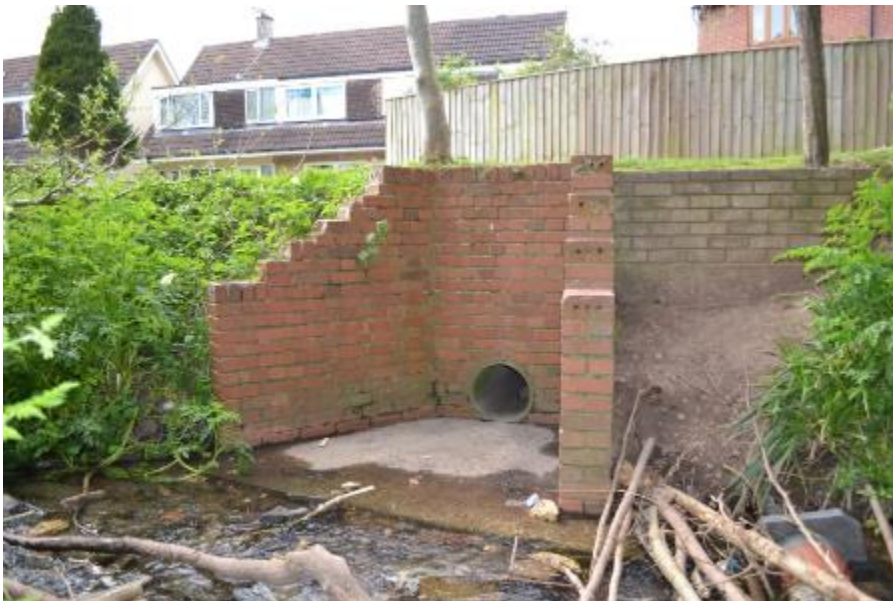
Figure 134: 30cm discharge pipe located on the right bank of St. Andrew's Stream 15m downstream from survey point SA8. No effluent was flowing from the pipe and no odour was present.
