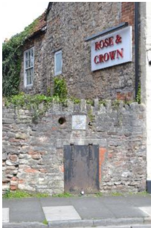
Figure 99: Wall at survey point SA2 behind which runs St. Andrew's Stream. The Stream runs from towards the pavement and is culverted from this point to survey point SA3
