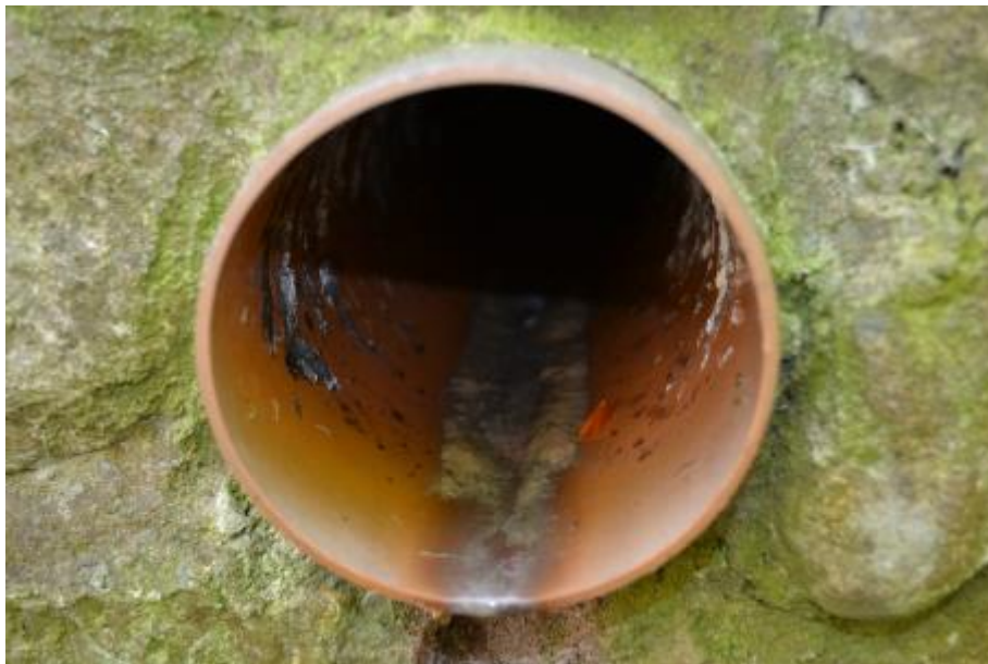
Figure 81: Close up view of the 15cm diameter pipe located on the left bank wall of Keward Brook at survey point KB17. Effluent is clearly visible in the pipe the pipe; a foul smelling odour was present.
