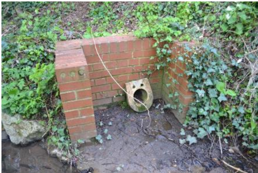
Figure 125: 10cm diameter discharge pipe located on the left bank of St. Andrew's Stream approximately 80m downstream from survey point SA7a. No effluent was flowing from the pipe and no odour was present.
