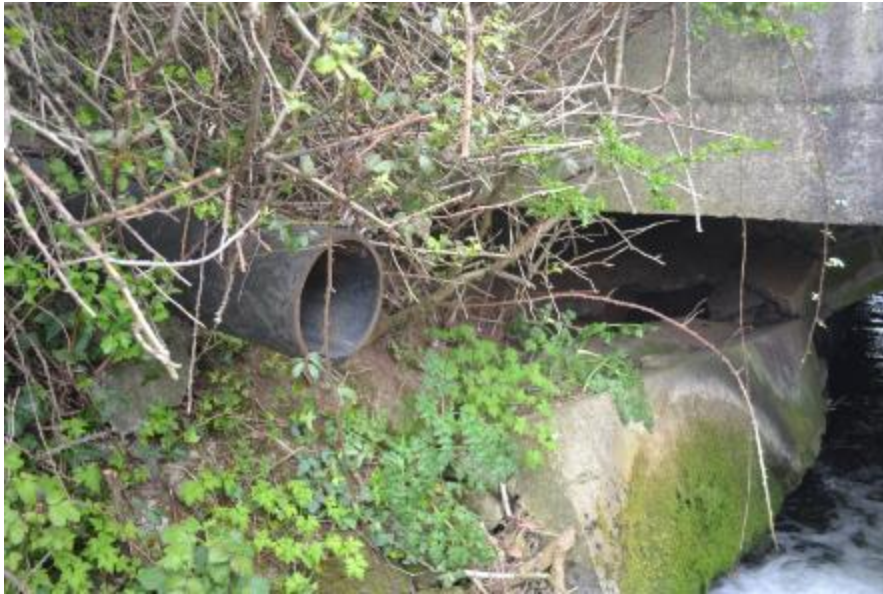
Figure 46: Discharge pipe located 10m downstream of survey point KB9 on the left bank. The 24cm diameter pipe was odourless and was not discharging effluent.
