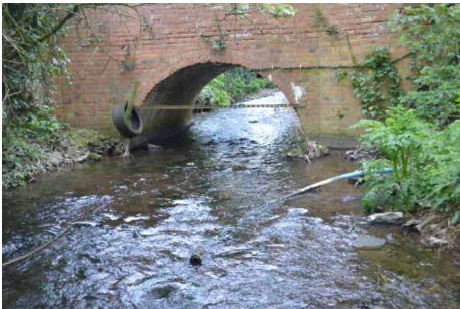
Figure 29: Upstream view of bridge approximately 15m downstream of survey point KB6. Note the metal bar running across the bridge arch, a stake supporting a tyre on the right bank (left in the image) and a blue pipe running into the stream.
