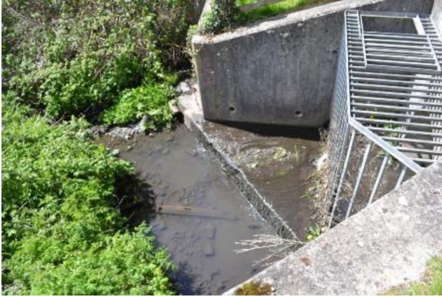
Figure 116: Culvert discharging water that passes through a screen filter at survey point SA6b. Litter is visible in the channel.
