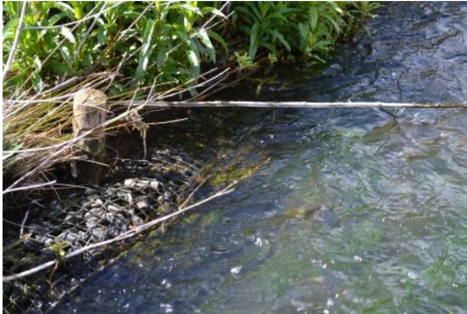
Figure 70: Rock and coir rolls placed situated along the left bank of Keward Brook, approximately 50m downstream from survey point KB15.
