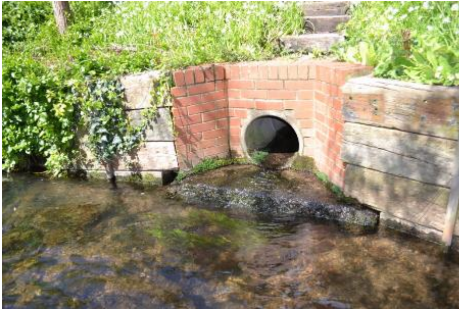
Figure 86: A 45cm diameter culvert pipe discharge pipe situated on the right bank of Keward Brook, approximately 75m downstream of survey point KB18. The pipe was discharging a constant flow of clear, odourless water, possibly flowing from St. Andrew's Stream.
