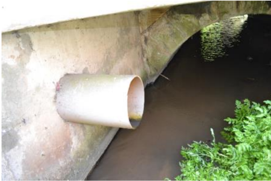
Figure 112: Discharge pipe located approximately 45m downstream of survey point SA5 on the left bank. The 30cm diameter pipe was odourless and was not discharging effluent.
