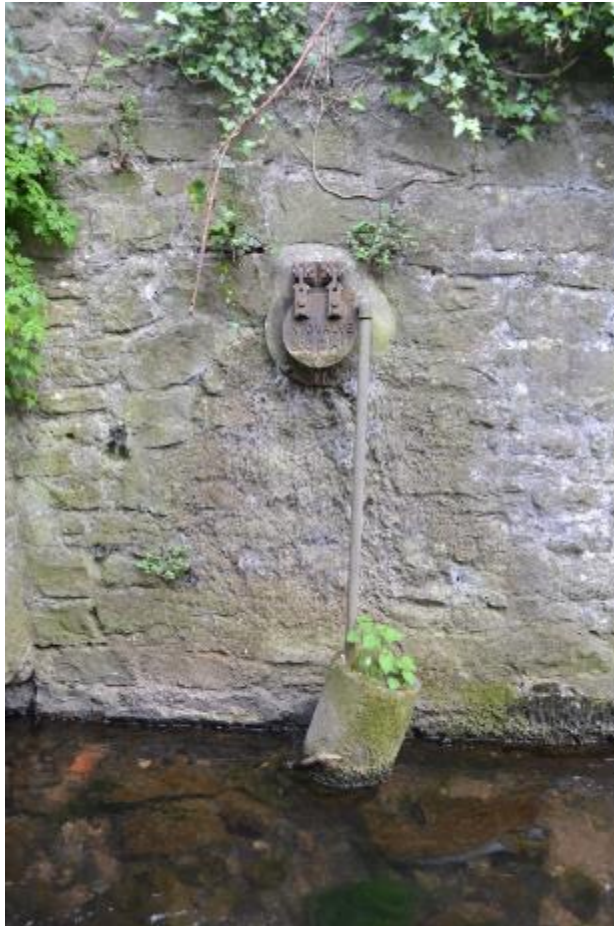
Figure 35: A 22cm diameter discharge pipe on the left bank at survey point KB7. No odour was present and no effluent was being discharged. Minimum staining is visible on the wall beneath the pipe.
